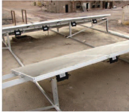
Images a&b: Two common sources of soiling: birds & sand
