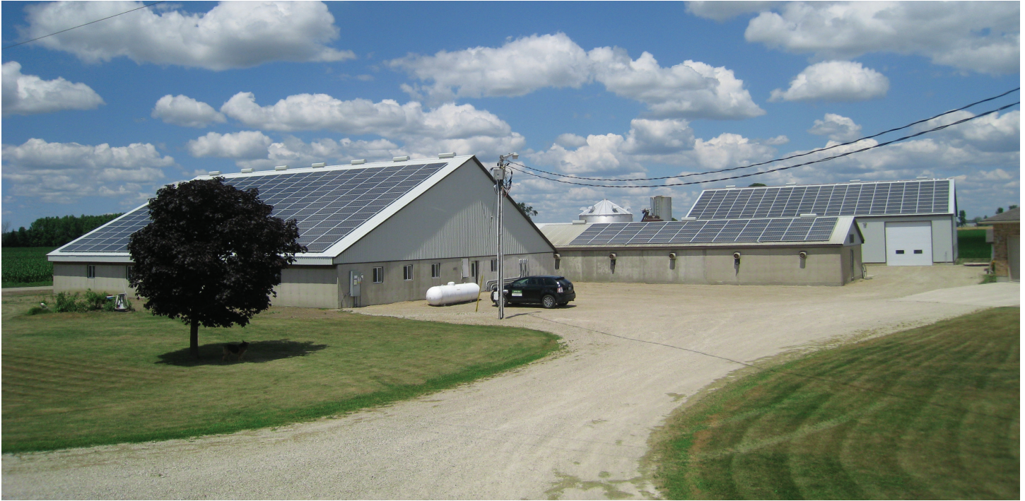
Figure 1: The Donkers installation in Monkton, Ontario - a 90kW harvest from three buildings. | Photo by Sashaan Solar
