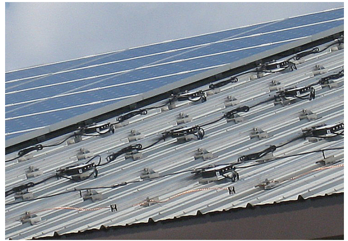
Figure 2: The SolarEdge power optimizers that harvest maximum energy from each module on the Donkers' barn. Photo by Sashaan Solar
